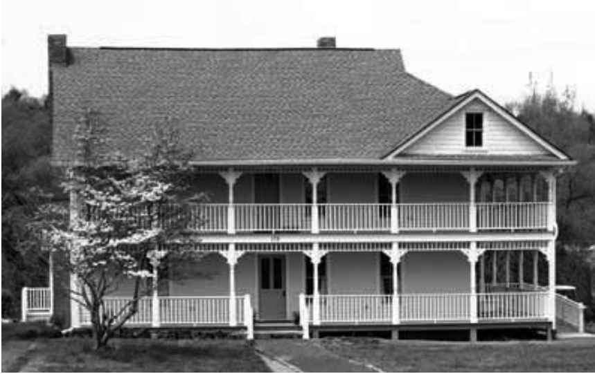
The Shook-Smathers House after renovation, 2005. Photo by Robin Hitch
